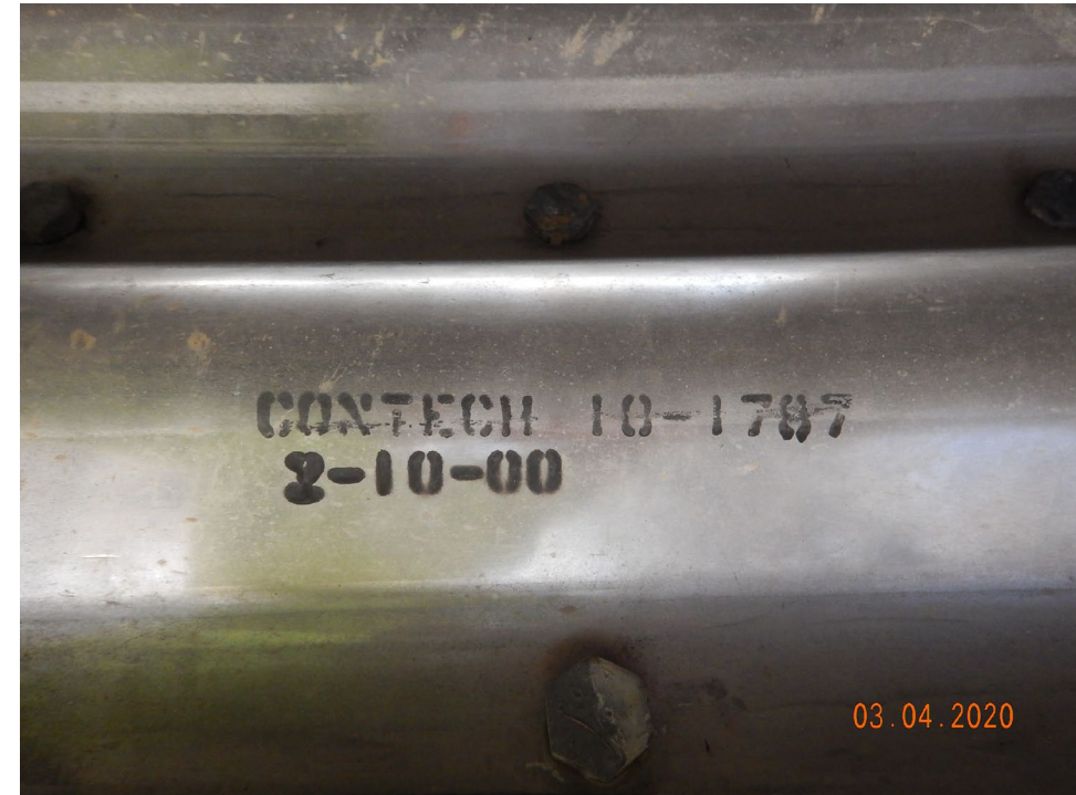
Photo showing structure stamp on underside of crown plate
