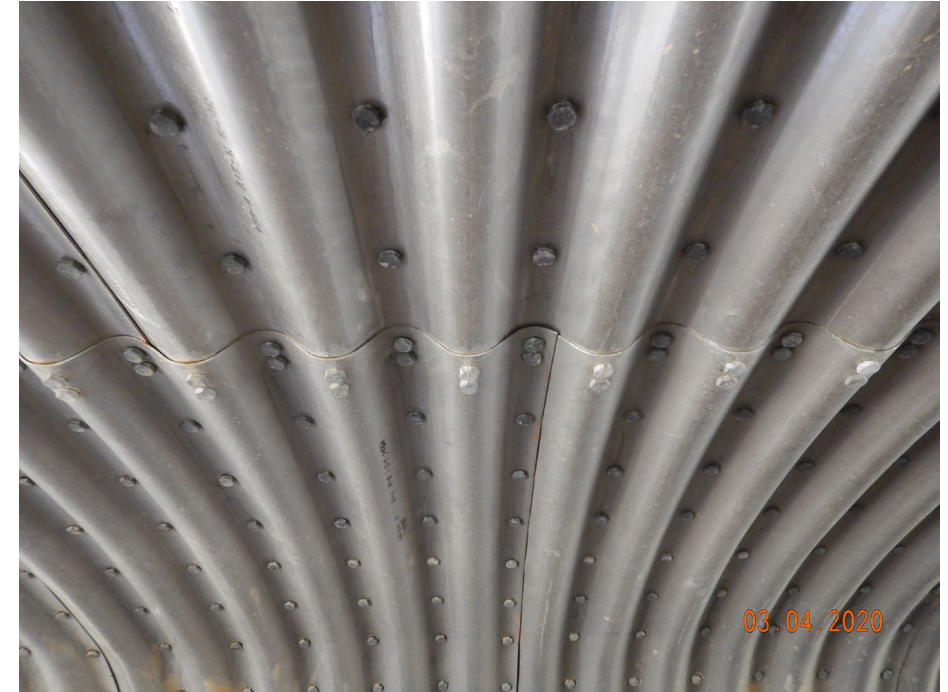
Photo showing rib bolt spacing in underside of structure
